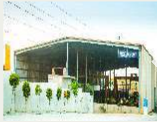
BCC PRECAST PLANT
